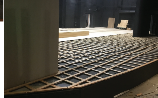
Kennesaw State University stage floor project featuring Harlequin WoodSpring and Harlequin Cascade.
